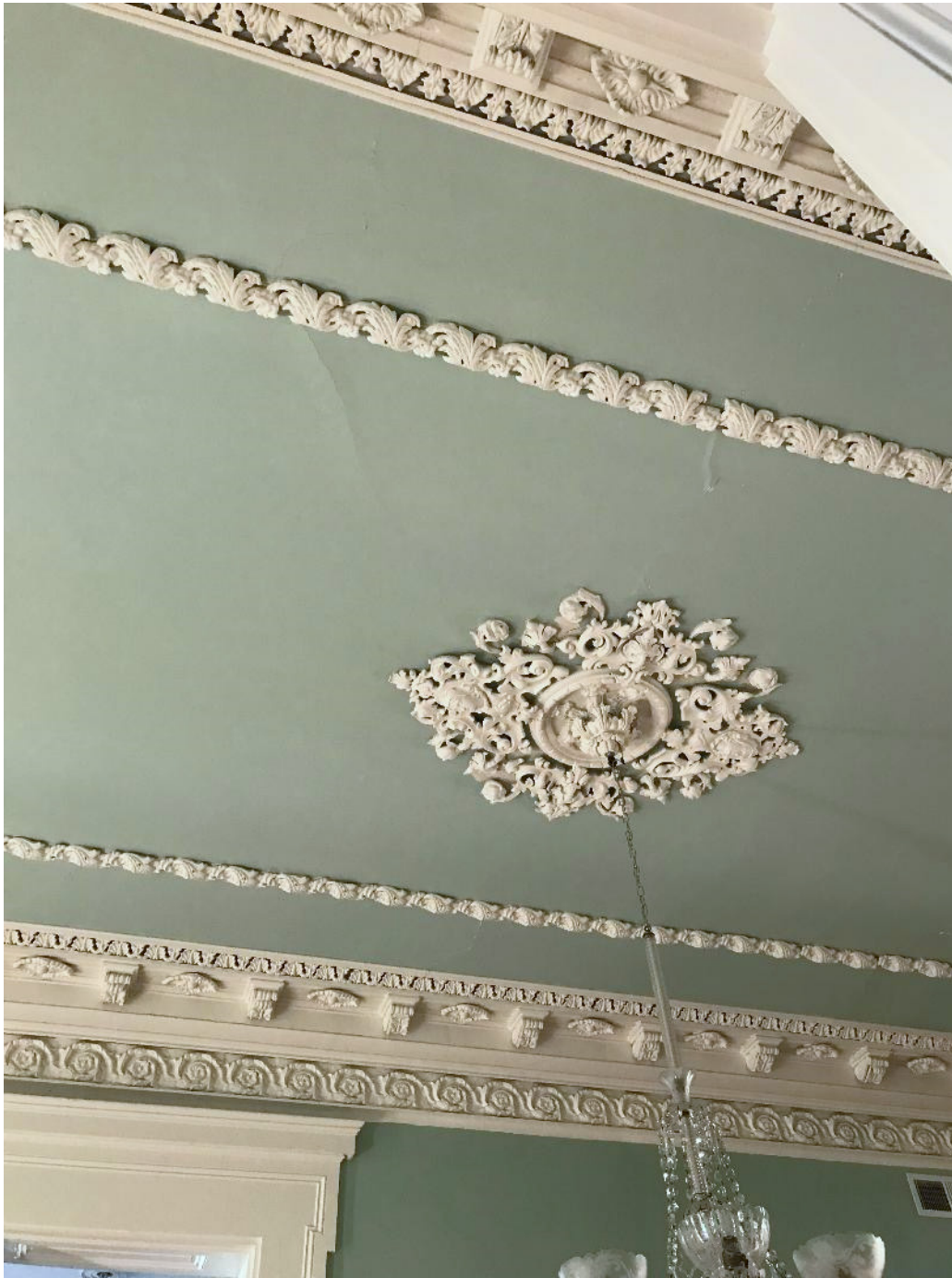
Original plaster medallion in the central hall. Photo courtesy of Peter W. Patout April 2018.
