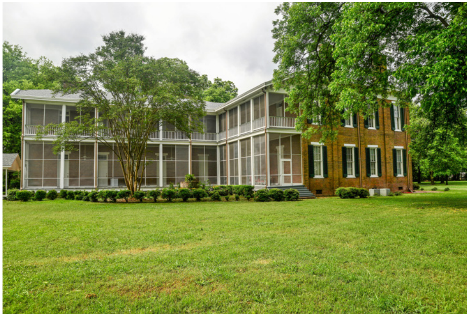
Two-story screened rear porch on south side of the mansion
